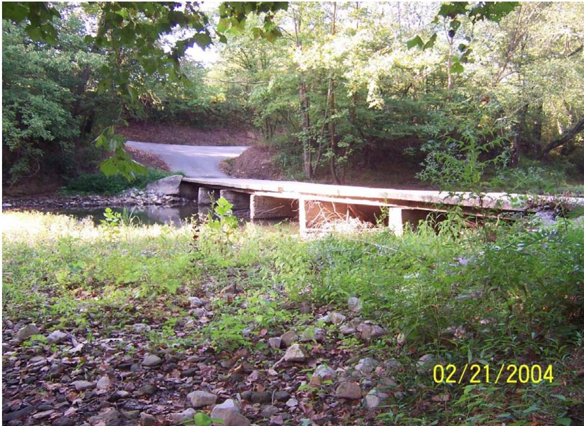
Exhibit 3: Sideview of Bridge
